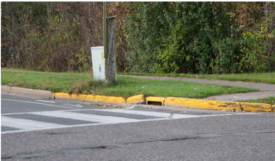
This is an example of an area along Broadway that is lacking curb cuts. Curb cuts make it easier for those with physical disabilities use these facilities.
