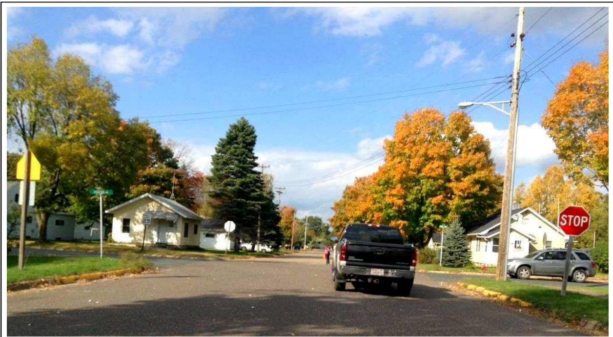
7 th Street facing north at the 7 th Street, Foster Avenue, and Park Avenue intersection.
