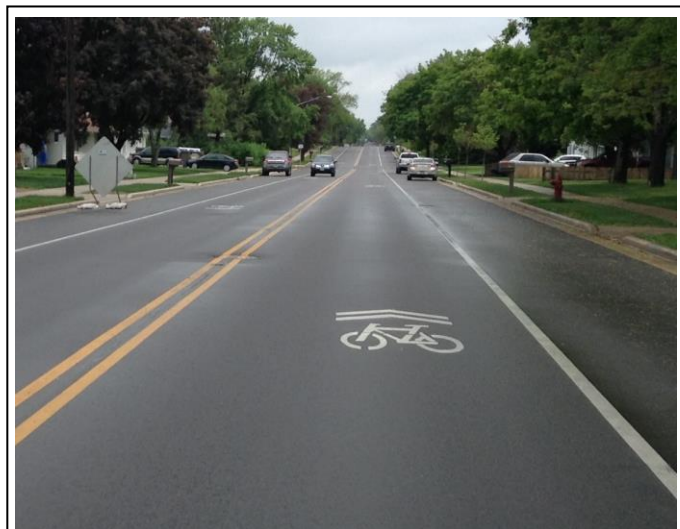
Example of a roadway with centerline, parking lines, and sharrows. Eau Claire, WI.
