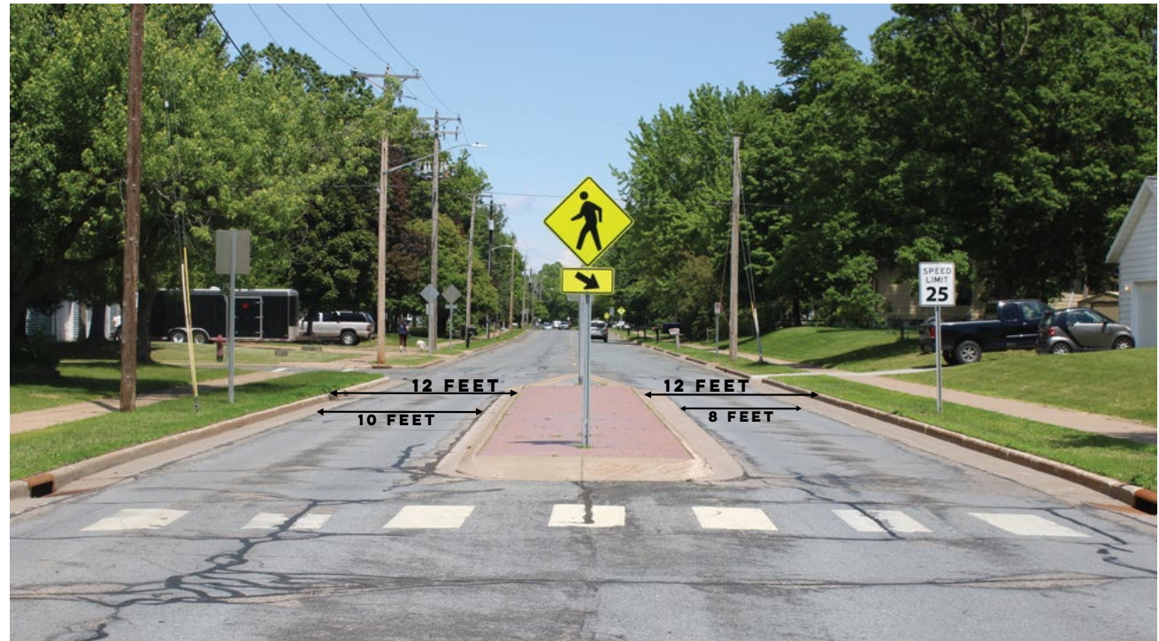
Eddy Lane Curb Pavement Extension Example
