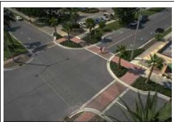
Pedestrian intersection with bump-outs. Source: FHWA
