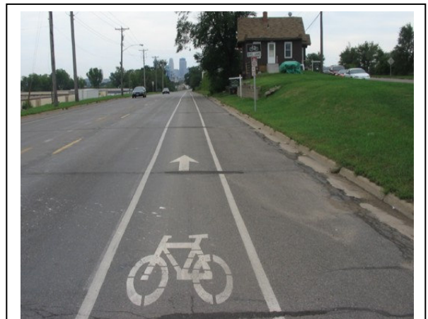
A bike lane outside of a parking lane. Source: City of Minneapolis, MN
